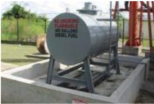
Figure 6: Bunding example 3
