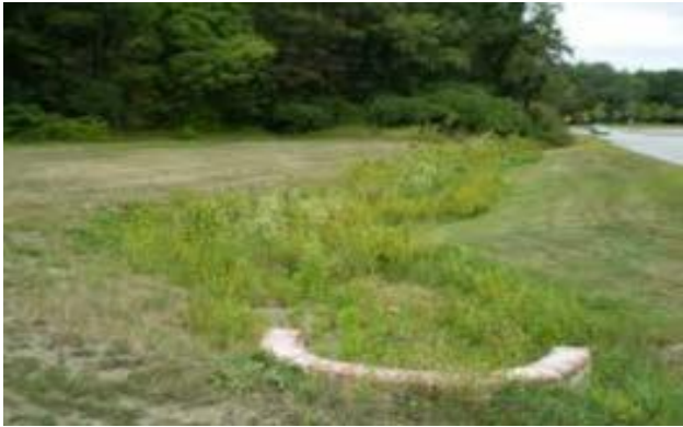
Figure 8: Grass filter strip
