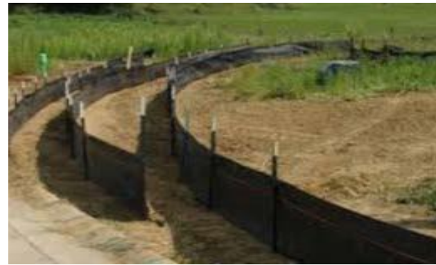
Figure 9: Proper placement of silt fencing for slopes
